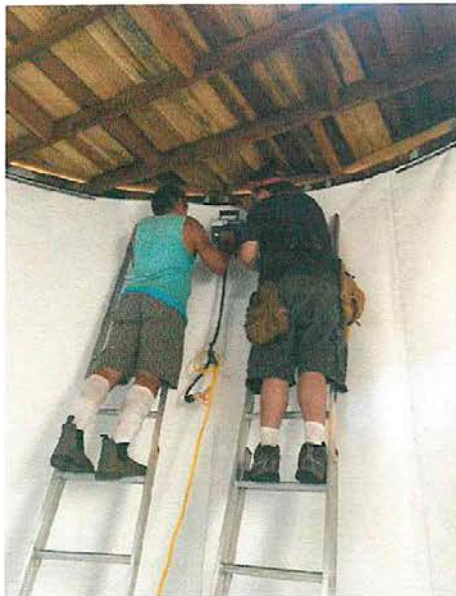
D. Moore & T. Moore wedge welding the wall panel together.
