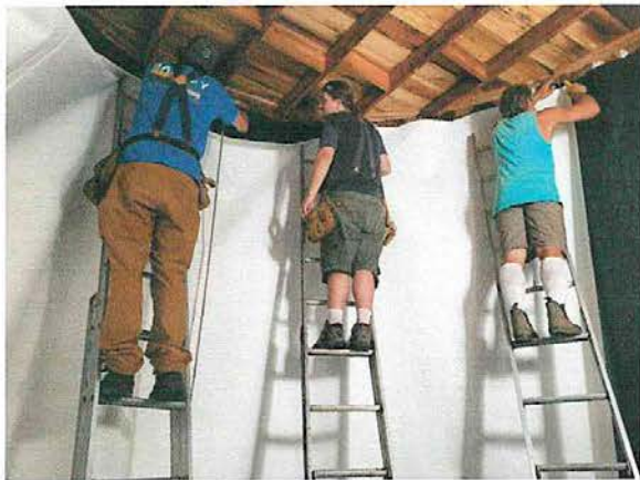
D. Moore, T. Moore & J. Burton hanging the wall panel.
