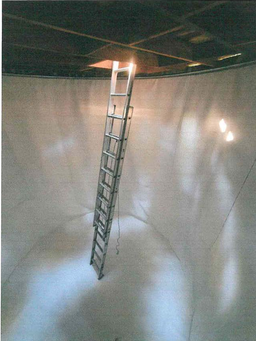
Pictured is the completed liner.
